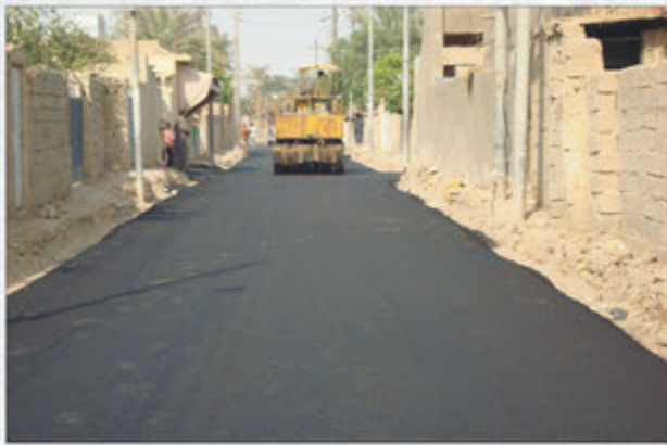
3.Paving streets Bour / Baghdad
